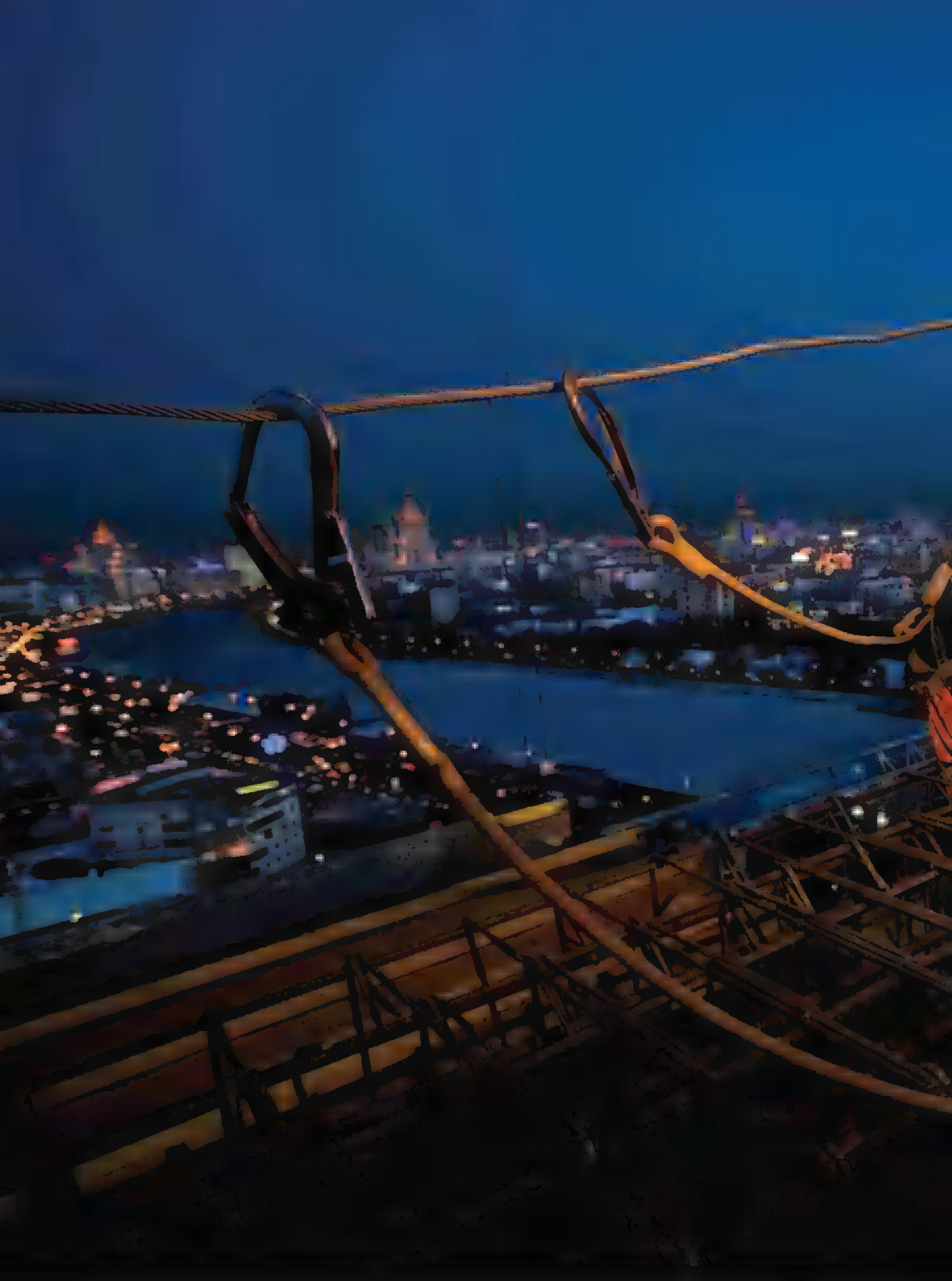
4:52 P.M. Darkness falls as a building rises along the Moscow River. Laborers, most from former Soviet republics,
